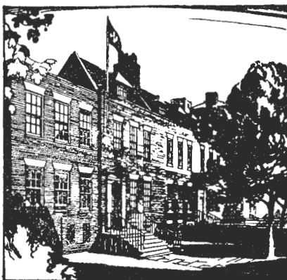
ROLAND HOUSE har facade mod Stepney Green.
